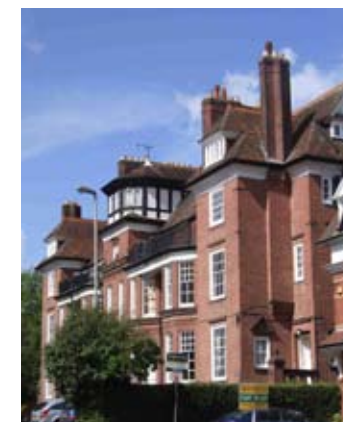
5. De Montfort Court, Stoneygate Road
