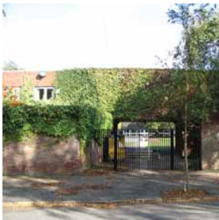
Digby Hall - Meadowcourt Road
